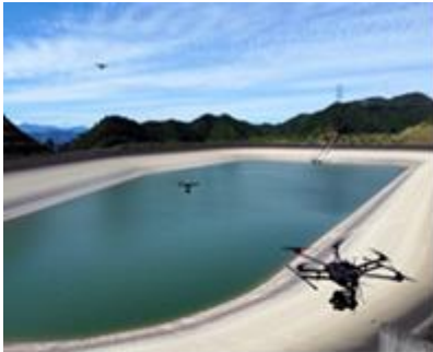
Image of dam impermeable wall taken by drone
