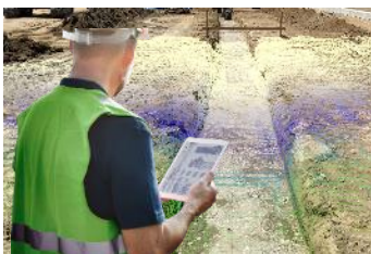
⑦ Construction surveying
